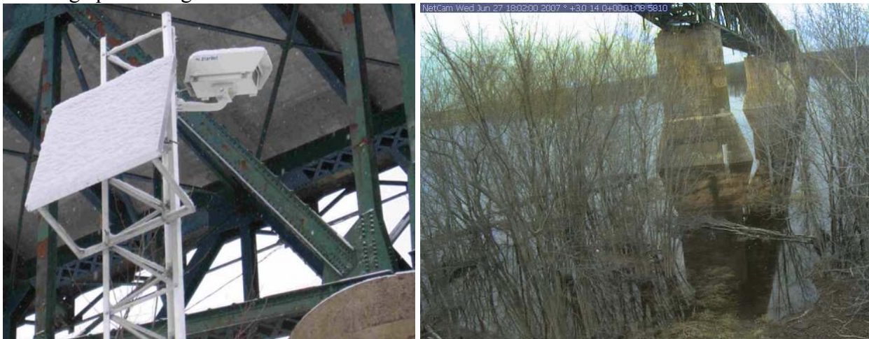
Figure 1: On the left is the cold weather camera (inside a weather-resistant enclosure) and solar panel on top of the 9 m high tower. The right image shows the camera view with a small focal length lens. The pier marker is visible slightly to the right of centre of the image.
